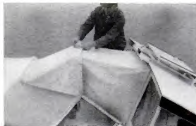
FINISHING TOUCHES are provided by the author in tying closed the little openings in mastlight seam
